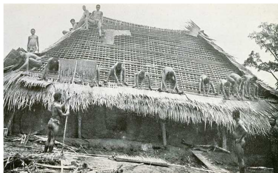
Figure 1.5: Thatching with palm leaf mats, among the Igbo people. Basden, G. T. Among the Ibos of Nigeria . Philadelphia: J.B. Lippincott, 1921, pg. 168.
